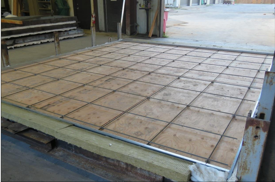
Figure B-3. Rebar Placed after Plywood Spline Added.
