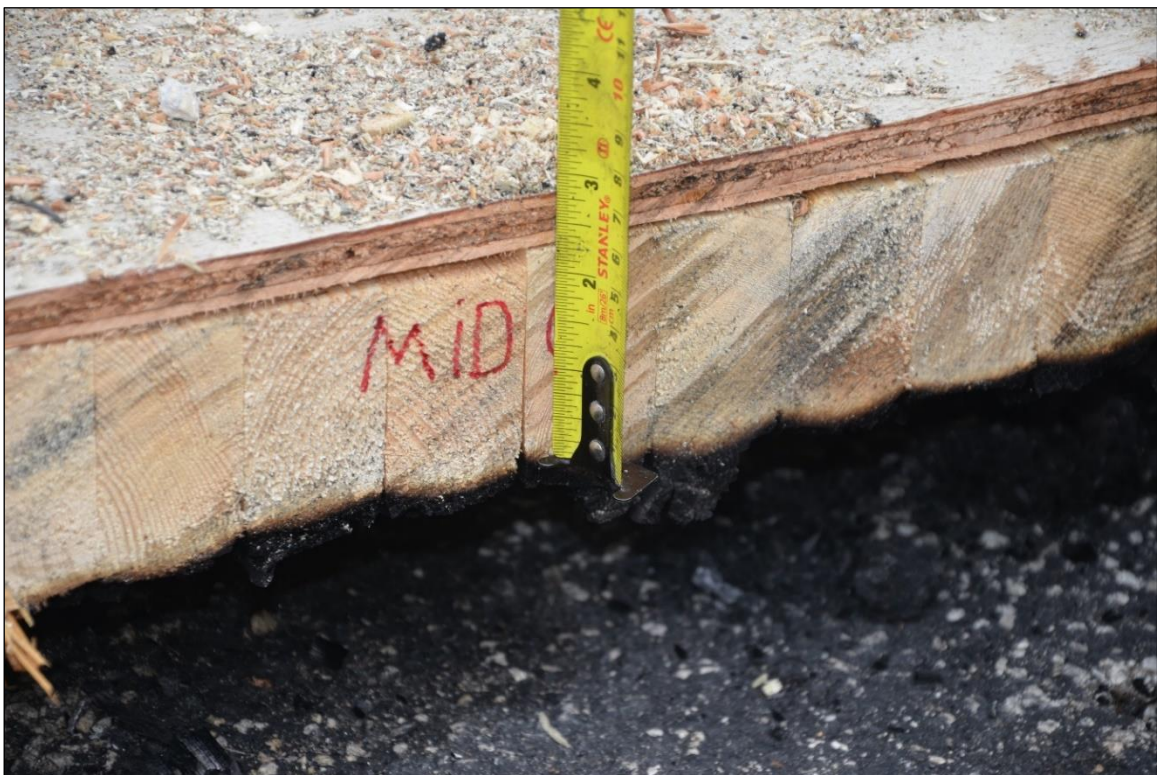
Figure B-12. Exposed Face Cross-Section of the Middle Quadrant after Cut.
